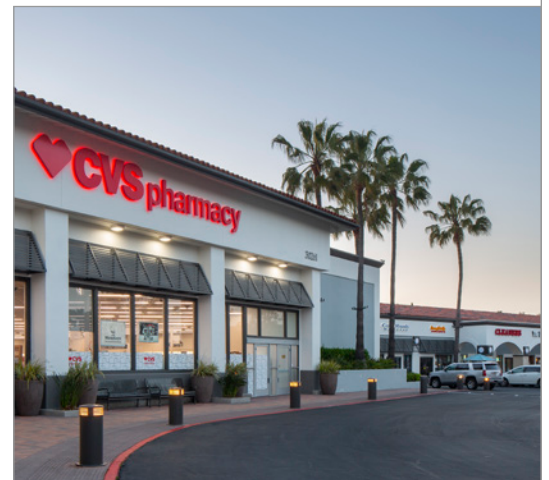
CVS/pharmacy, one of center's anchors.
