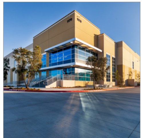
Shea Center West Corona industrial center.
