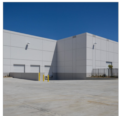
Loading docks at 17332 Gothard
