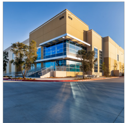
Shea Center West Corona industrial center.
